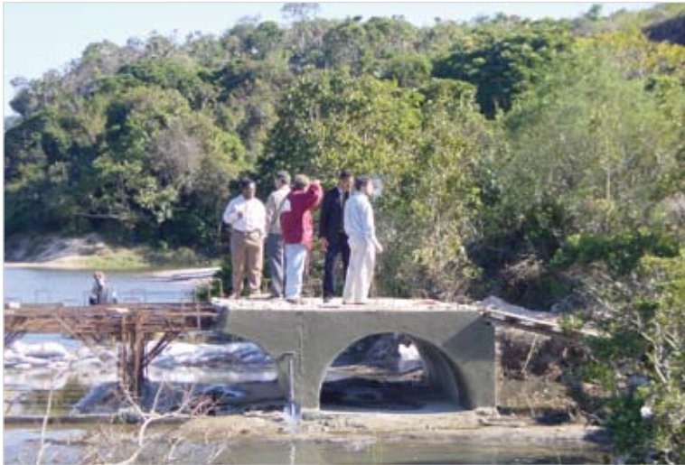
Photo 5.1: Initial construction showing the reinforcement and a cast arch
