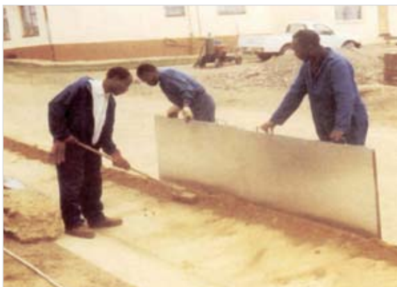
Photo 4.17: Protection of kerbs, drains, etc.
