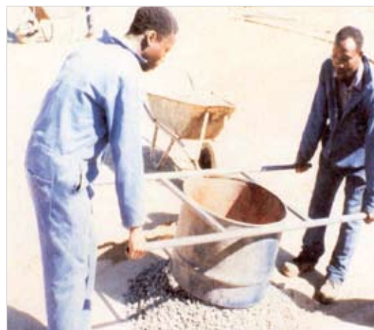
Photos 4.13 and 4.14: Spotting of aggregate
