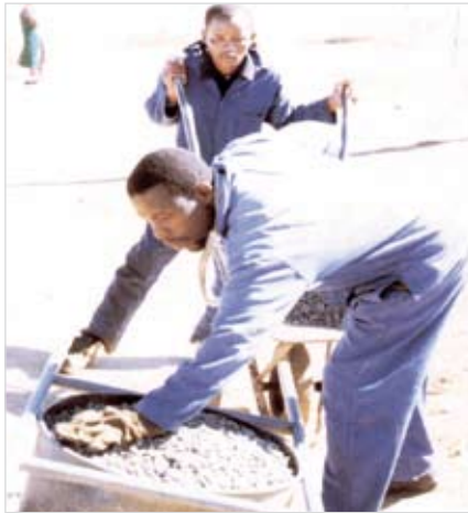
Photos 4.33 and 4.34: Spotting of aggregate
