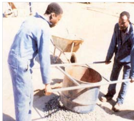
Photos 4.46 and 4.47: Spotting of aggregate
