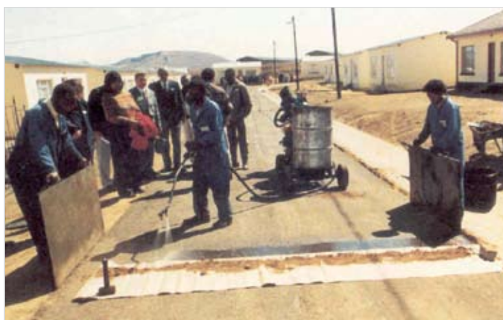
Photo 4.6: Spraying with motorised hand sprayer with screens and reinforced paper in use
