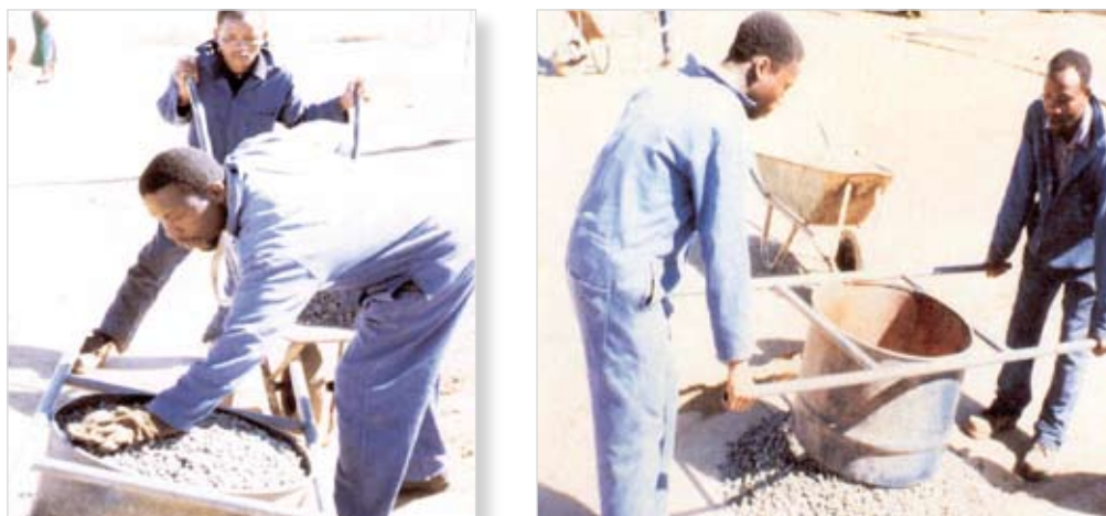
Photos 4.9 and 4.10: Spotting of aggregate
