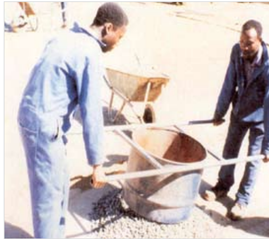
Photos 4.33 and 4.34: Spotting of aggregate
