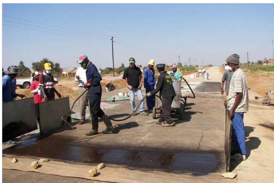
Photo 4.2: Spraying using protective screens and reinforced paper
