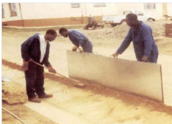
Photo 4.7: Protection of kerbs, drains etc.
