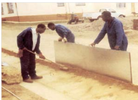
Photo 4.30: Protection of kerbs, drains etc.
