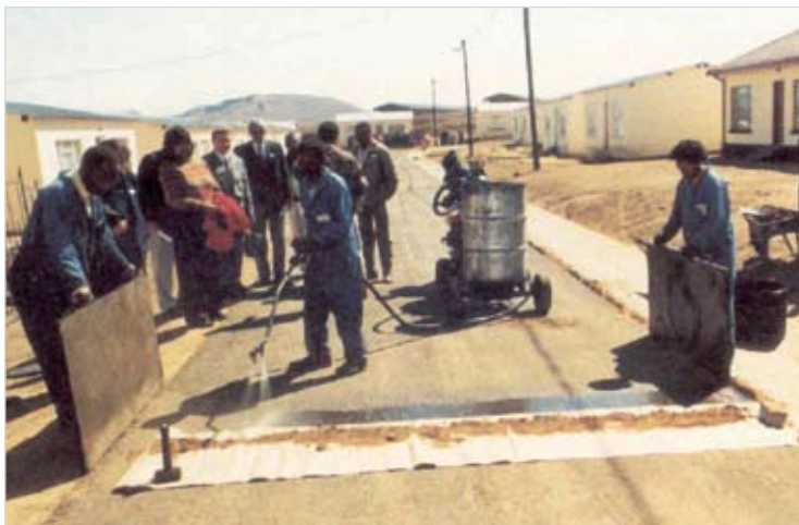
Photo 4.29: Spraying operation using motorised hand sprayer, with screens and reinforced paper in place
