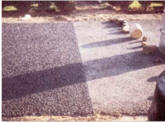
Photo 4.31: Neat construction joint due to use of reinforced paper
