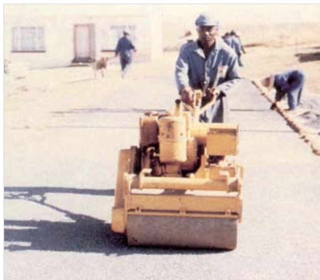
Photo 4.35: Compaction of the aggregate
