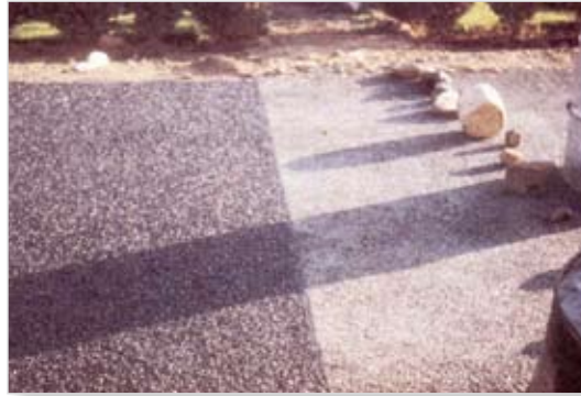
Photo 4.8: Neat construction joint due to use of reinforced paper
