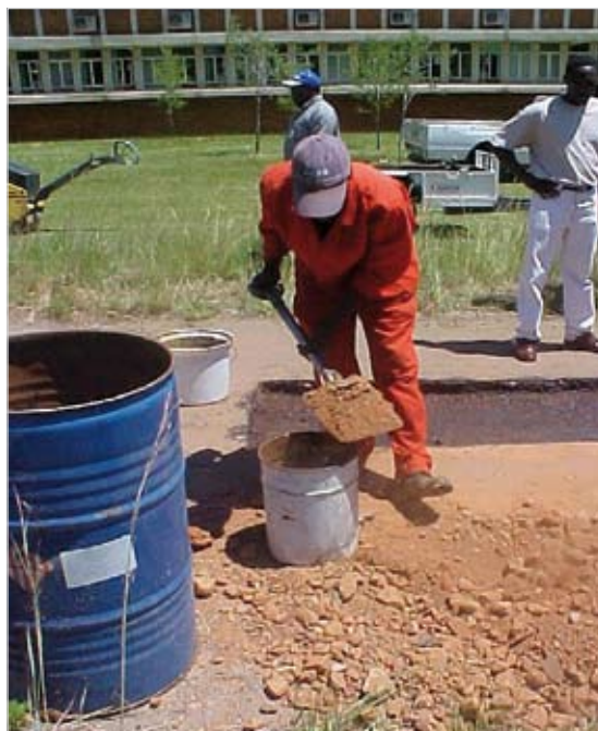
Photo 3.2: Measure aggregate
