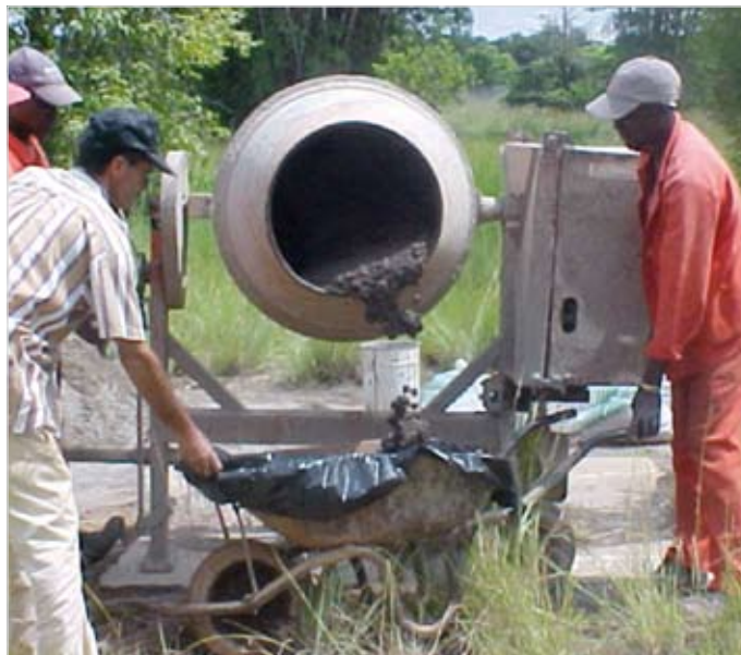
Photo 3.14: Discharge into wheelbarrows
