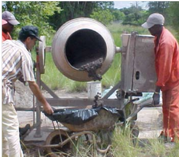
Photo 3.7: Discharge into wheelbarrows
