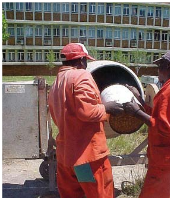
Photo 3.10: Add aggregate and cement
