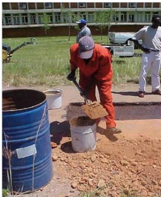
Photo 3.9: Measure aggregate
