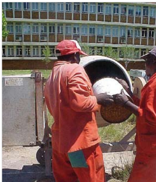
Photo 3.3: Add aggregate and cement
